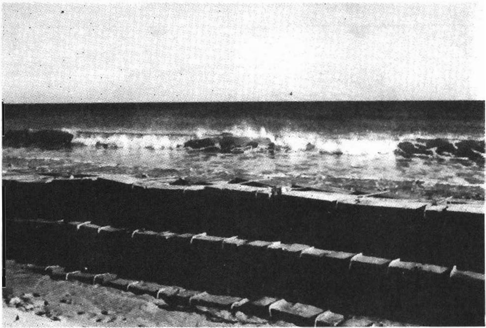
Fig. 131 - A concrete block ("sandgrabber") perched beach at Duxbury Spit, MA.
