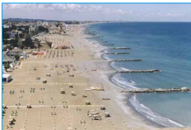
Figure 105. Misano Adriatico: 1600 m long stretch defended by 26 groynes. Between 1983 and 2007, 876,000 m 3 of sand were carried to this stretch of coast.
