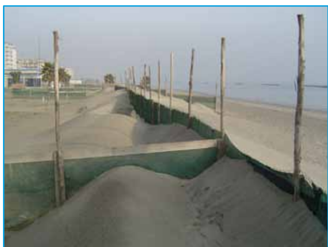
Figure 85 - permanent windbreak barrier 2 years after its construction (Porto Garibaldi beach). Please note the formation of a stable dune on the left side
