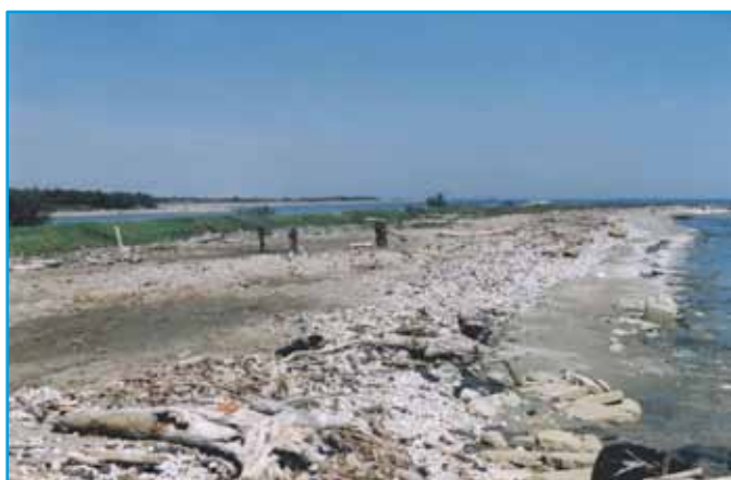
Figure 108. The remains of the defense works destroyed by sea along the first 500 m stretch south of the Reno river mouth.
