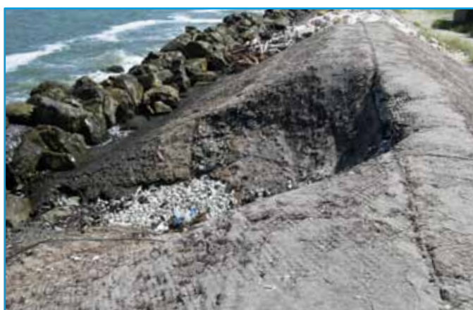
Figure 109 - The riprap lining close to the military shooting range, along a 3 km long stretch, is subject to continuous collapses due to frequent sea overflows.
