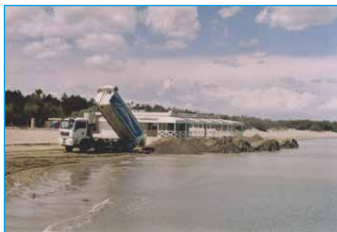
Figure 90 - Beach nourishment by means of sand from land-based quarries undoubtedly is the solution with the heaviest environmental impact
