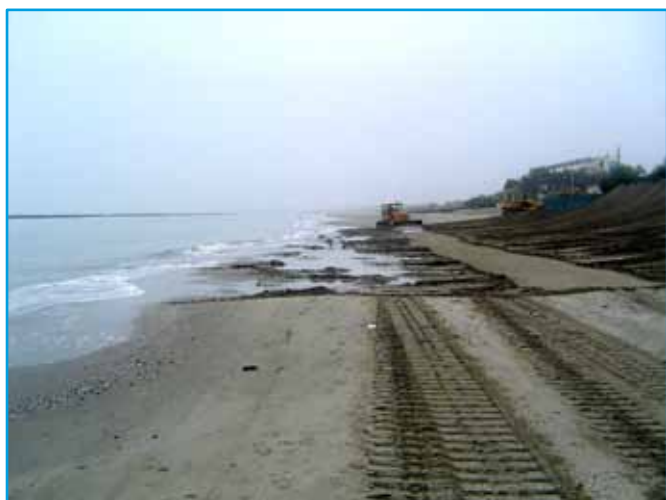
Figure 83. Left: not properly built winter defence embankment, by removing the sand from the foreshore. Right: properly built winter defence embankment, with sand coming from other sources and with the right shape
